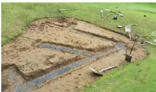
Marking out installation (10.00 am)
