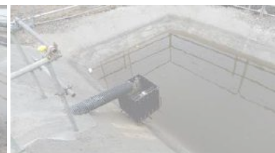
The final discharge through a Smart Sponge® Ultra Urban Filter was tested by the EA.
